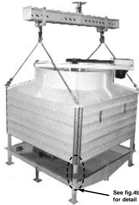
Figure 4a - Joining Casing to Pan section
